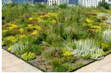
Figure 29: Semi-intensive green roof (Accredited Green Roof Professional, n.d.)
